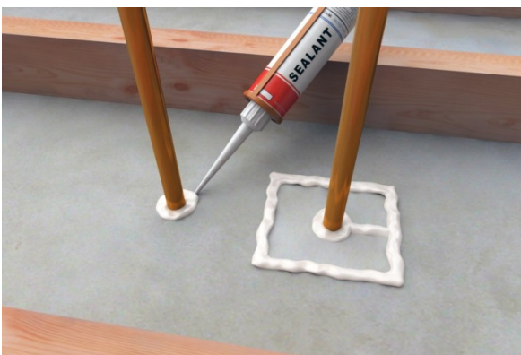
Figure 1: Sealing of Perforations Through Plasterboard Ceiling
