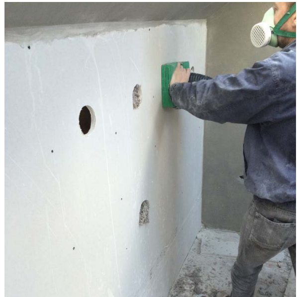
Figure 4: Operative pumping insulation into timber framed wall
