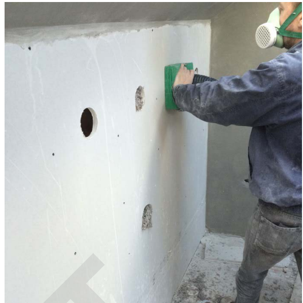
Figure 4: Operative pumping insulation into timber framed wall
